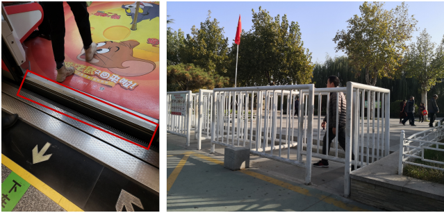
Figure 3: (Left) Local subway system has a gap of over 100 mm between the train and the platform which can decrease the accessibility of the subway system to wheelchair users; (Right) the entrance gate of a park blocks wheelchair users.
